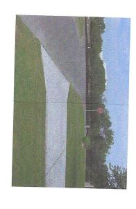
**Dip Style Driveway**Used when the roadside ditch is less than 12" deep.
